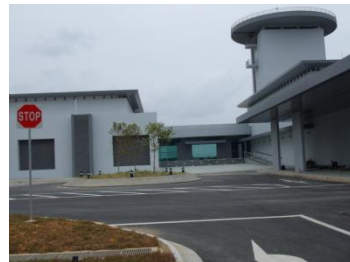
LORADS III building
